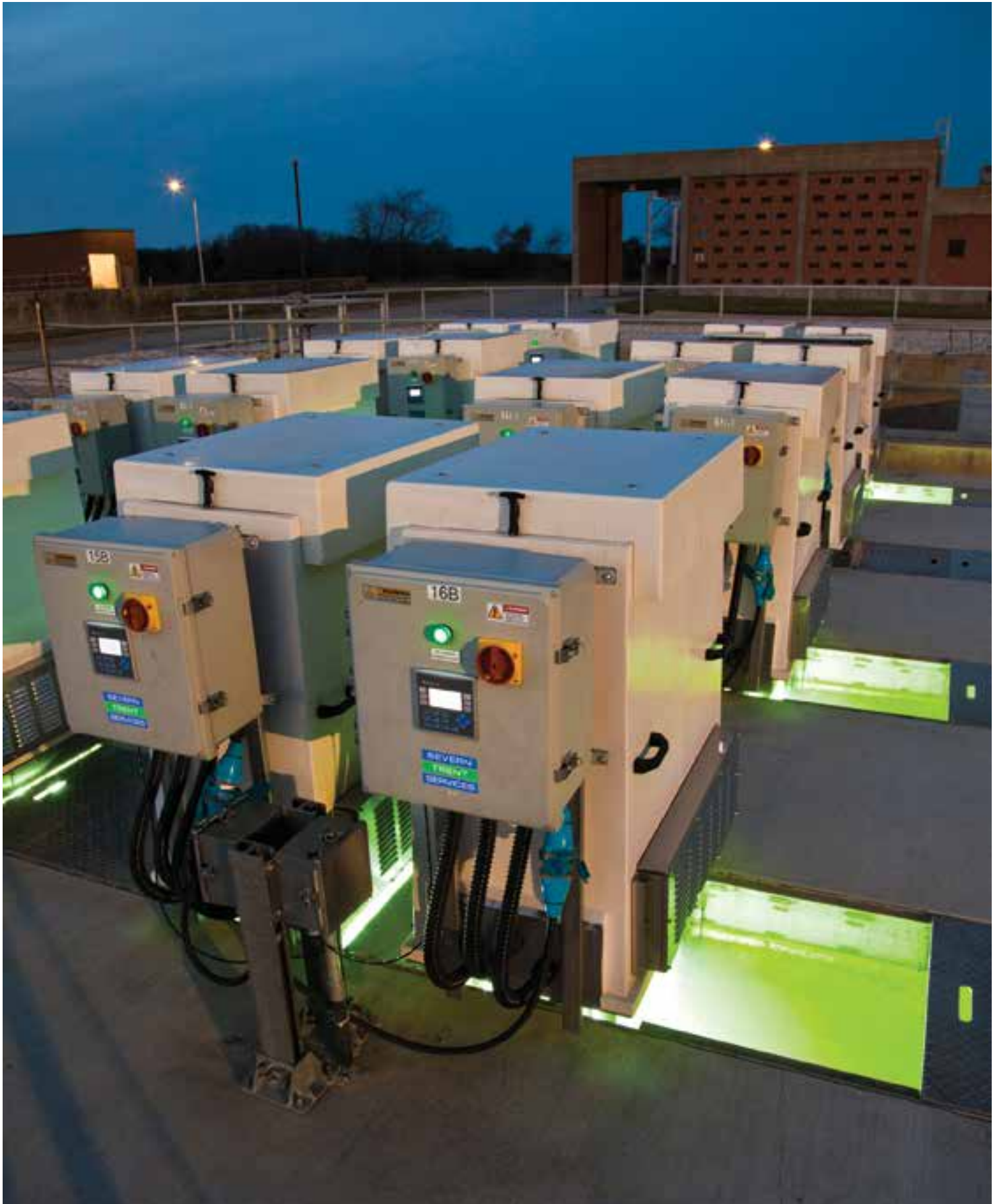
MicroDynamics® OCS 660 Open Channel Microwave UV Disinfection at Kent County, Delaware, USA
