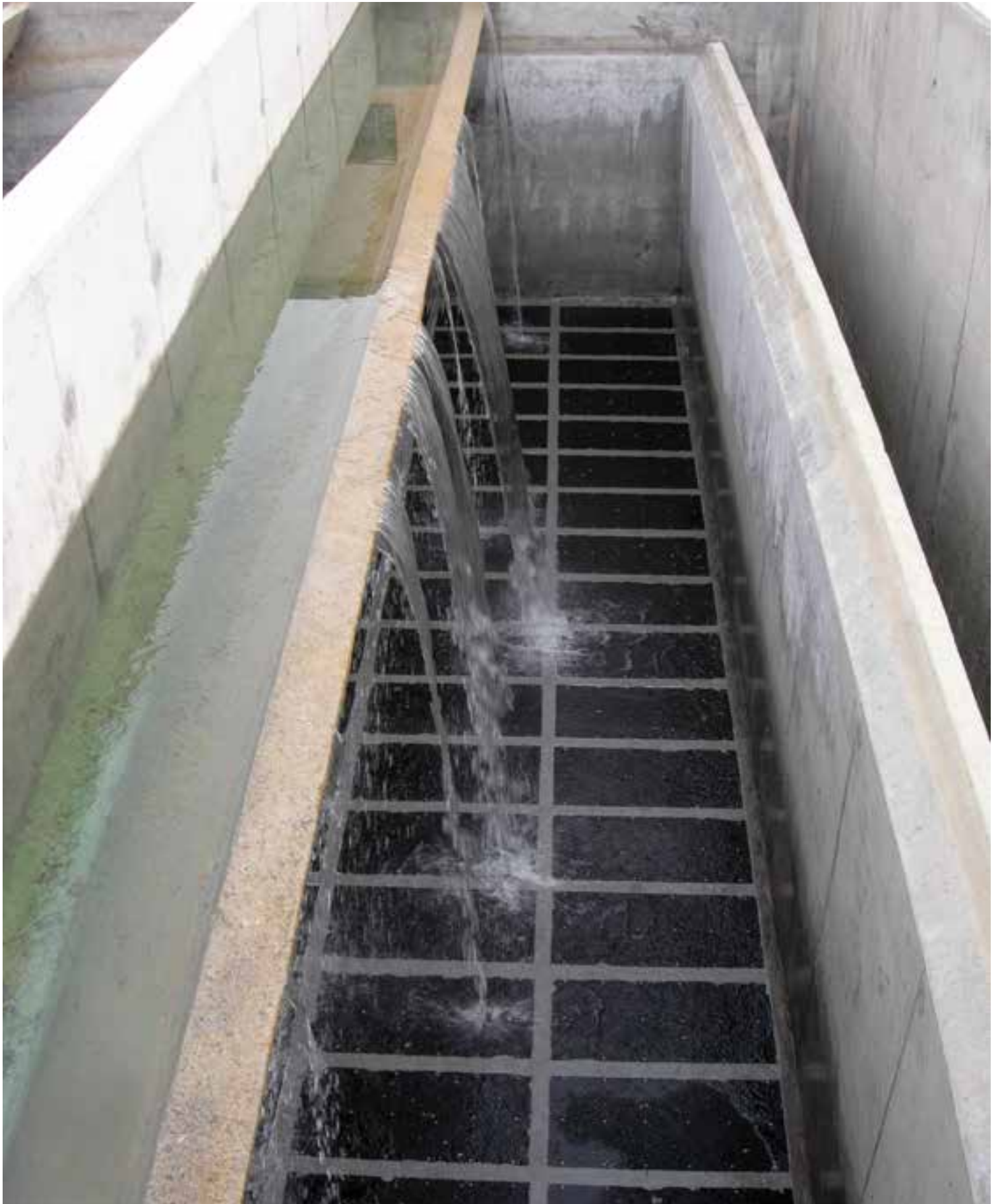
TETRA® LP Block™ Dual Parallel Lateral Underdrain Filters
