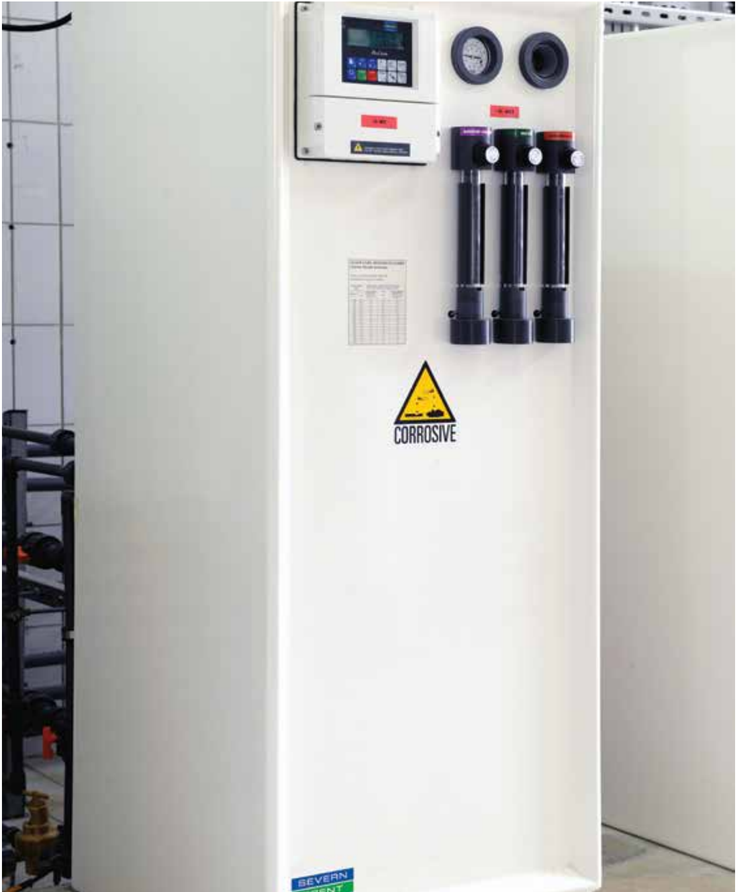
Capital Controls® G4000 Chlorine Dioxide Generator — Dubai, UAE
