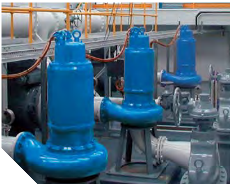
Wastewater pumping station with submersible pumps in dry mode
